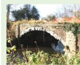
Within half a mile of the Nynehead drive aqueduct the GWC crossed over the Tone on another of James Green's cast-iron troughed aqueducts. Although the side plates are similarly splayed, in this case the bottom plates are flat. The towpath on one side and a track on the other were carried by
