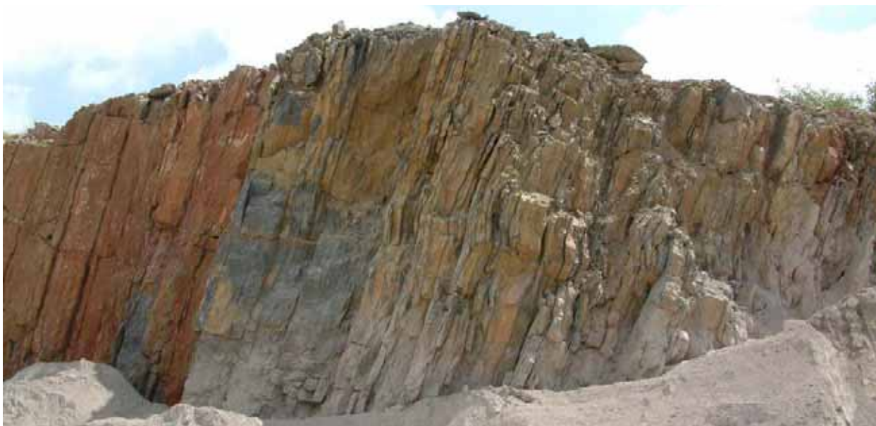
Photo PO 8 Halecombe Quarry, Loc 06 Junction between Lower Limestone Shale to the right and Black Rock Limestone to the left. Grid Ref ST70460 47223 c171mAOD Photo ref HA-06a Facing East
